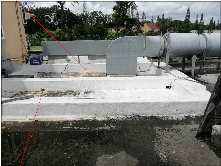
EXISTING HOLES TO UPSTAND BEAMS TO BE WIDENED AND 110mm PVC PIPE TO BE EPOXY GROUTED
