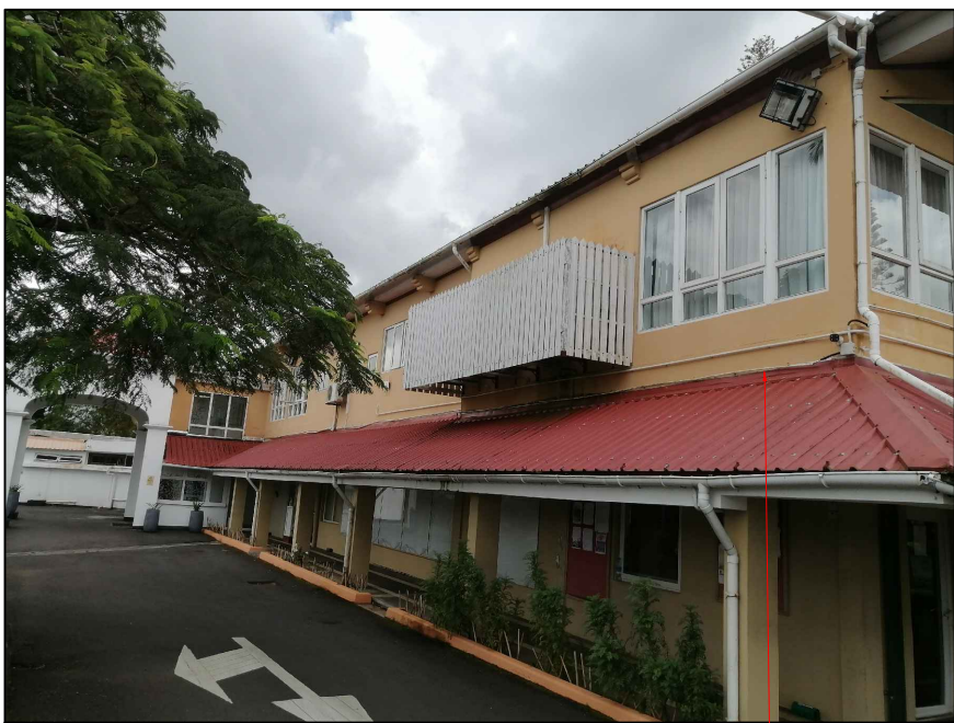
NEW WATERPROOFING TO METAL SHEETING TO BE PROVIDED COMPLETE WITH FLASHING (NEAR CADDY MASTER OFFICE) TO ENGINEER'S ACCEPTANCE
