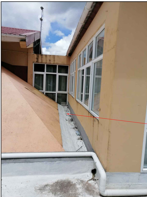
NEW WATERPROOFING TO METAL SHEETING TO BE PROVIDED COMPLETE WITH FLASHING (NEAR CADDY MASTER OFFICE) TO ENGINEER'S ACCEPTANCE
