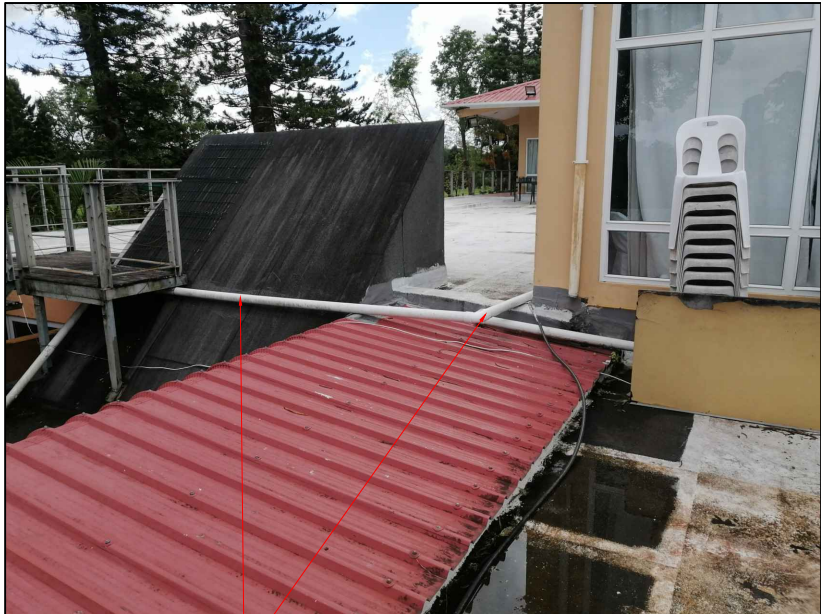
EXISTING RAINWATER PIPES TO BE REDONE AND REDIRECTED TO SOAKAWAY AT GARDEN
