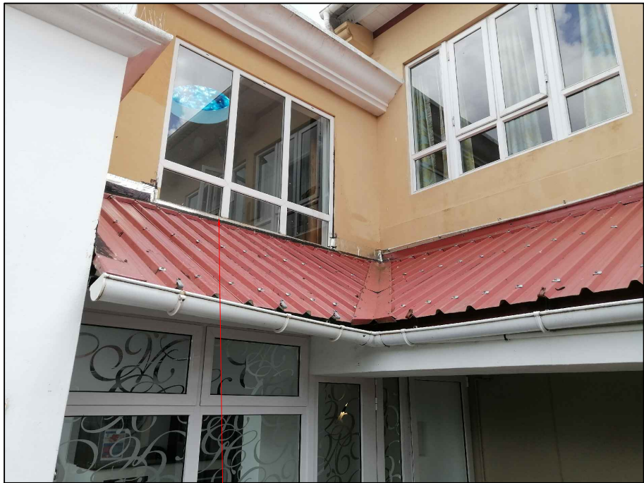
EXISTING WATERPROOFING TO METAL SHEETING TO BE REMOVED AND NEW TO BE DONE COMPLETE WITH FLASHING (NEAR RECEPTION AREA) TO ENGINEER'S ACCEPTANCE
