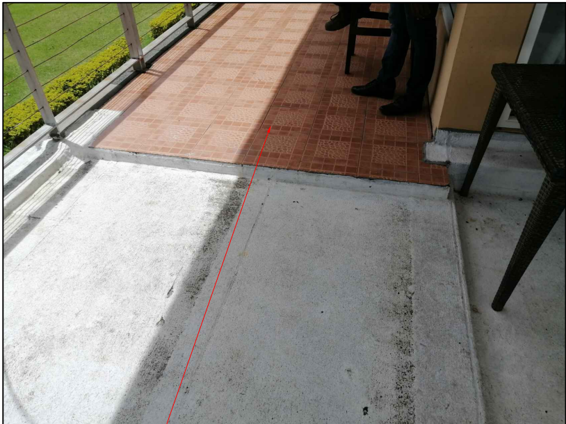
EXISTING TILES TO BE REMOVED, EXPANSION JOINT TO BE RE DONE NEW WATERPROOFING TO COVER EXPANSION JOINT (ABOVE RESTAURANT)
